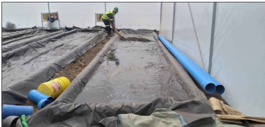
Fig. 2 Emptying Faecal sludge to the greenhouse for drying
